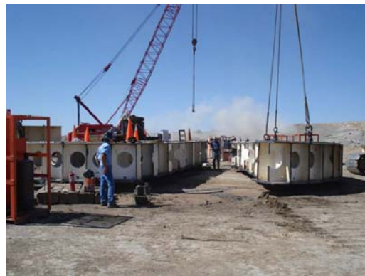
Final Disassembly of Dragline
