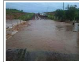
Flooded access to the Isaac Plains coal mine.
