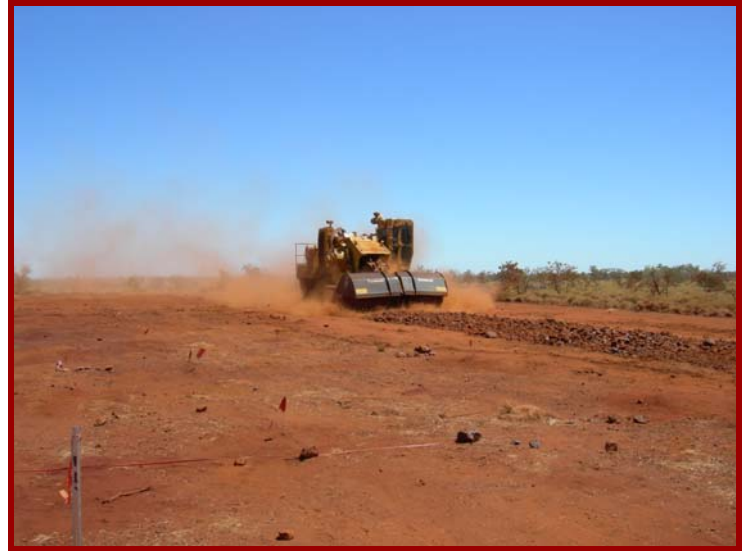
Continuous Miner at Upper Cane Bulk Sample Site
