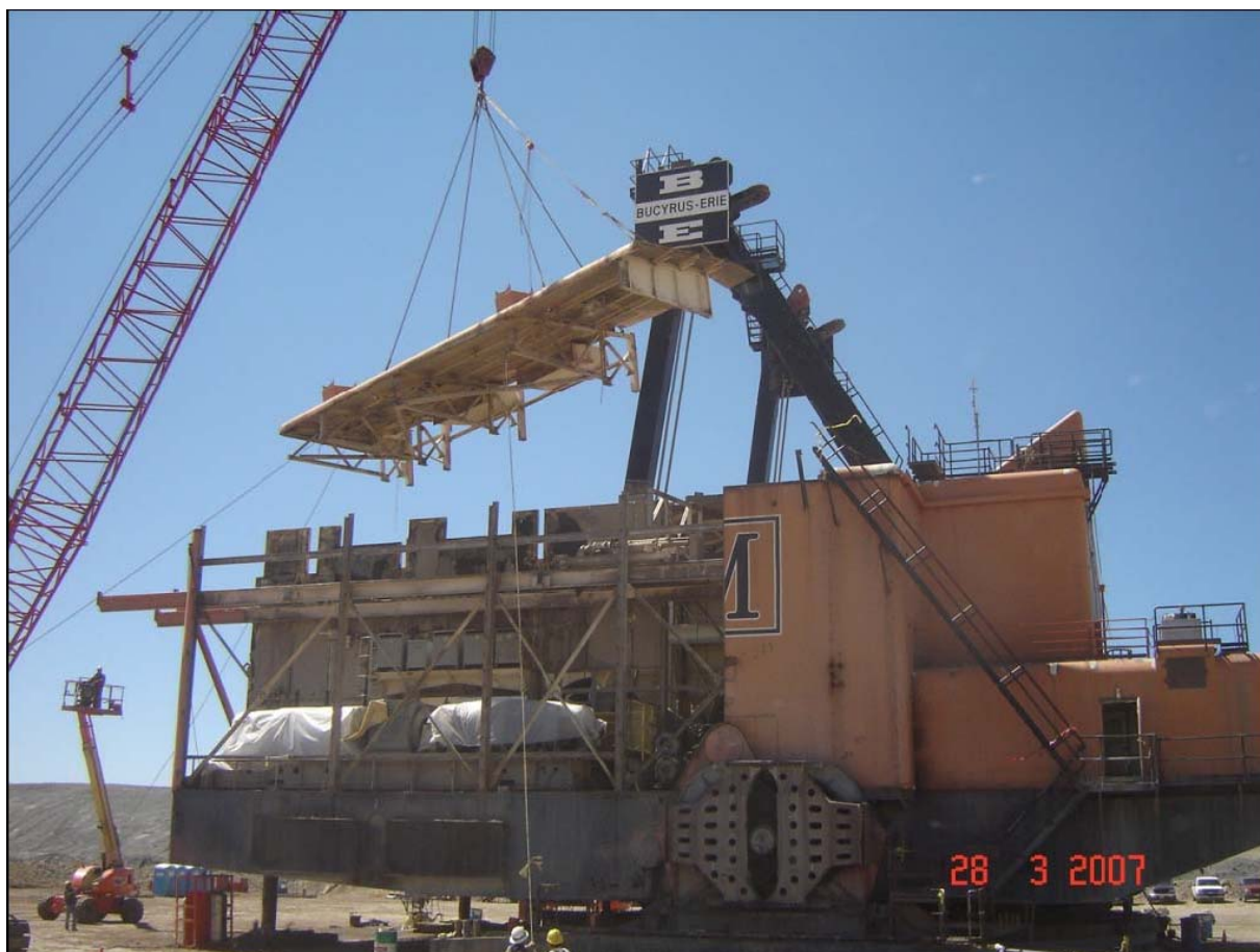
Removal of dragline roof section
